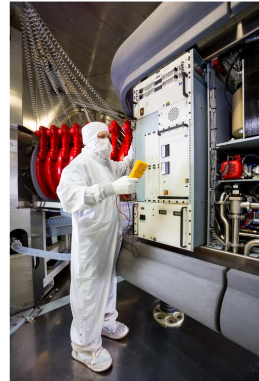
Picture of preventive maintenance work on an Implant tool
